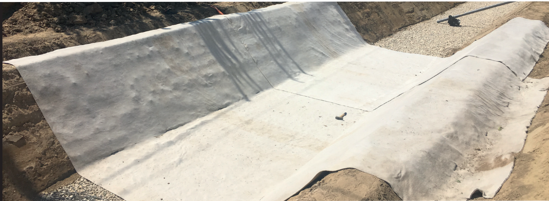
CANAL AND DITCH LINING
